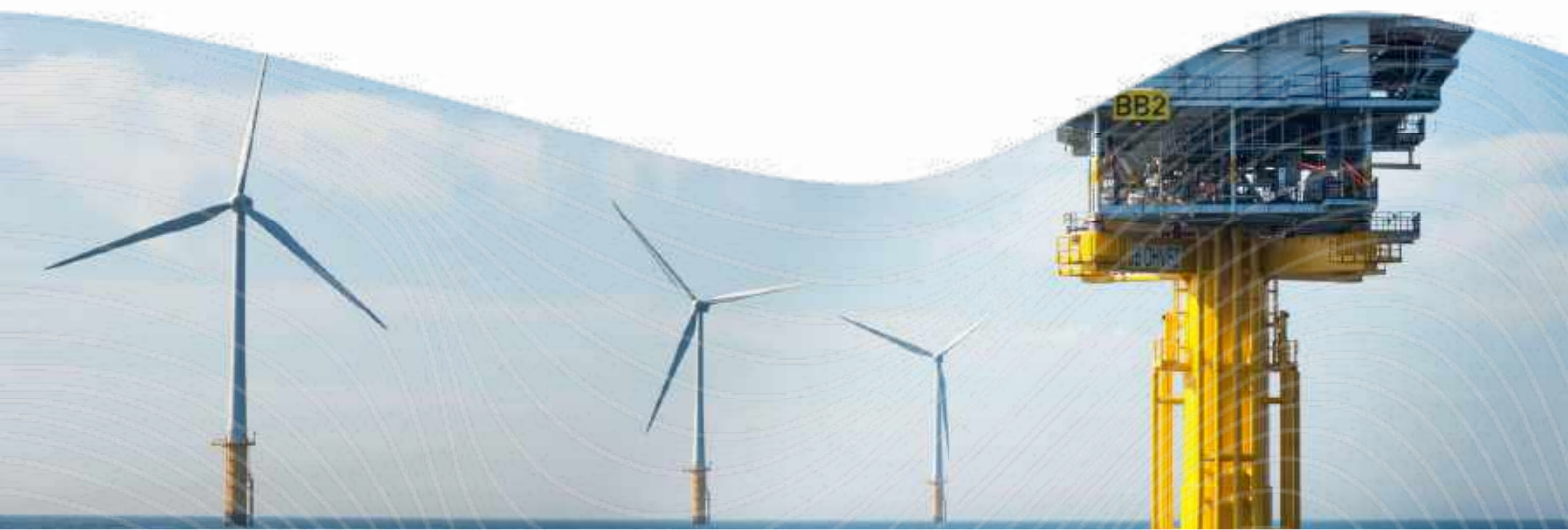
Image: Offshore High Voltage Station, Nobelwind, Belgian North Sea, Courtesy of Parkwind
